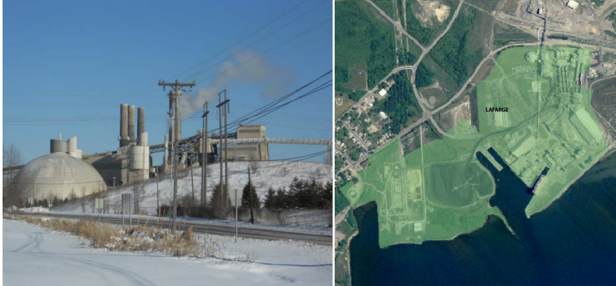
Figure 5-15 LaFarge Cement Plant & Arial View of Property
