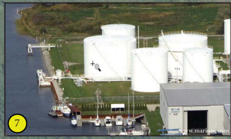
View of the US Oil bulk storage facility located just north of Walstrom Marine. Notice the the easy access for docking and small amount of useable land currently available.
