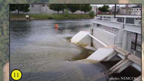
11 View of the dam located just south of the tissue company. The spillway is located directly below this and there is sidewalk to provide circulation and good views of the river.
