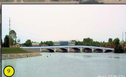
9 View looking south towards the Lincoln Avenue bridge. The stone seawall looks to be in good condition and fits in the surroundings very well.
