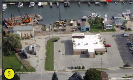
View of Ryba Marine Const. from above looking east towards the marina. Notice the close proximity of the working dock to the residential use to the south.
