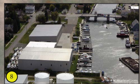
View looking south at the facilities of Walstrom Marine. Notice the constraint of the channel width at this point due to the uses on both sides of the river.
