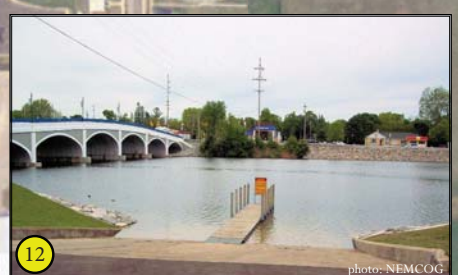
12 View looking west from the Lincoln Street Boat Access Site at two public boat ramps south of the dam and boat lock..
