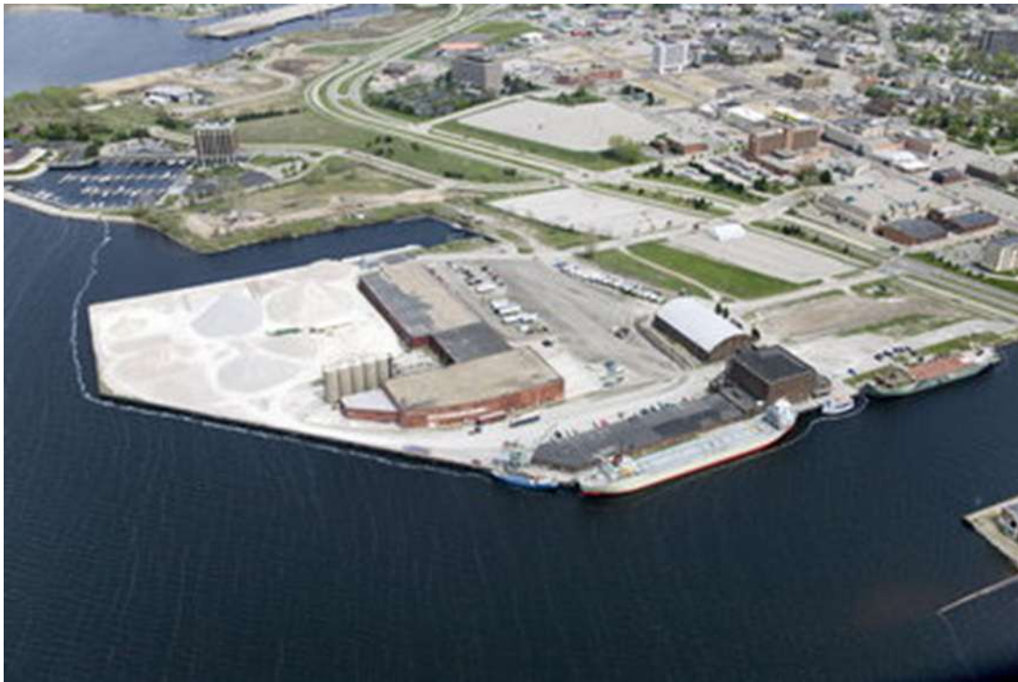
Figure 12-6 Birds eye view of the ports major loading dock and the Terrace Point Marina, Port of Muskegon
