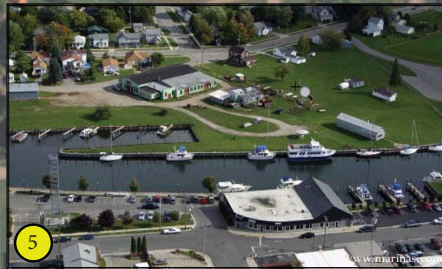
5 View looking east toward the Cheboygan Harbor Marina, which is located just north of East Park & presents pedestrian circulation opportunities.
