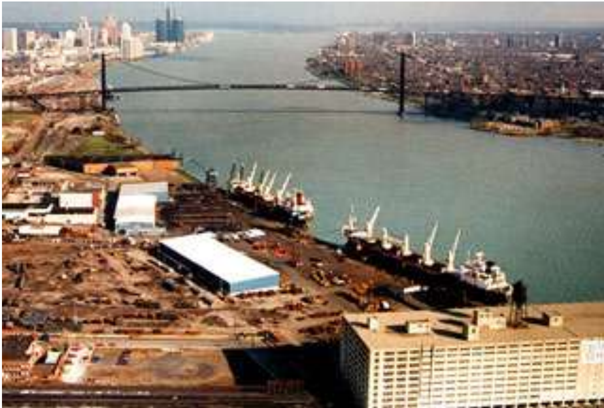
Figure 12-2 Picture demonstrating the use of one of the many terminals found in the 32 mile stretch of the Detroit River that is included in the Port Authorities jurisdiction
