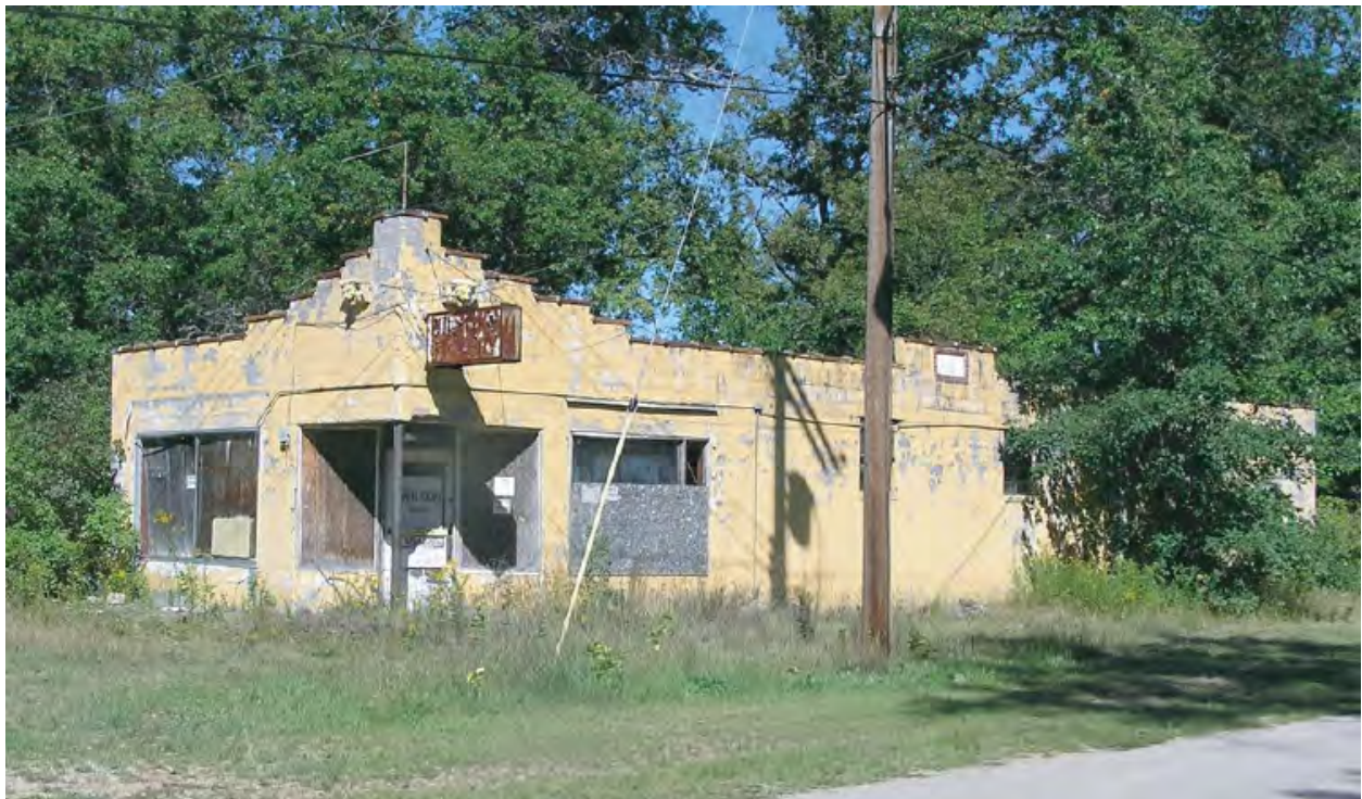
Figure 17: Example of Commercial Building and Concrete Block Structure: Wilson’s Grocery, 332 E. Wilson Drive (Vacant). Cultural Resource Management Plan, 2009.
