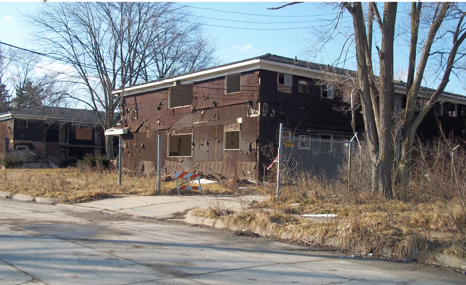
Abandoned Homes on St. Mary's St.
