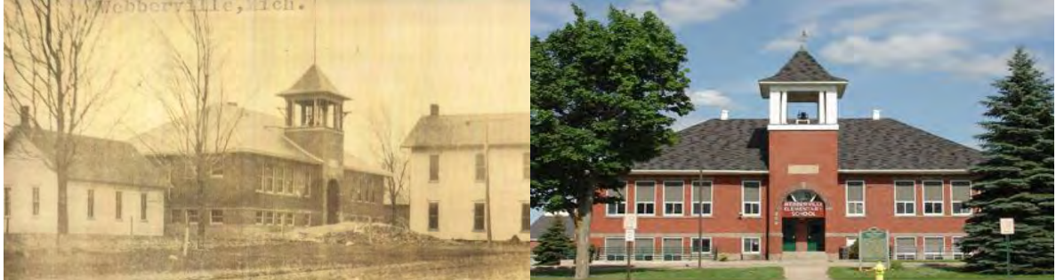
Figures 1.4 & 1.5. Webberville Elementary School, 1913 (left) & 2010 (right)
