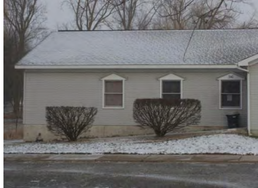
Figure 2.19. “Good” Condition Parcel
