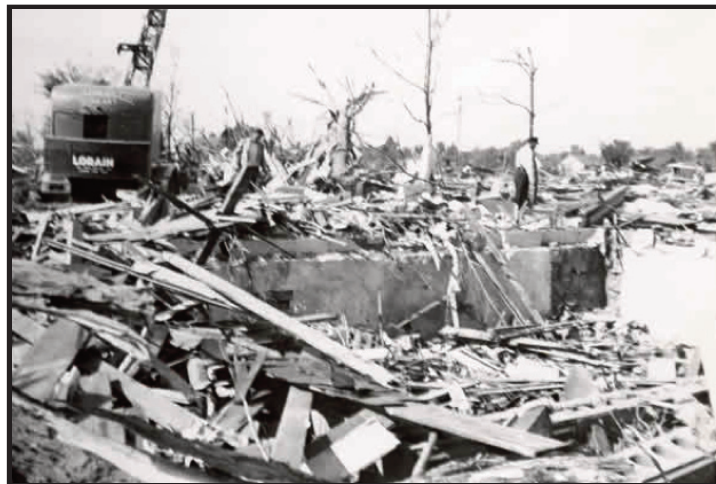
Figure 2.3.1: Flint Tornado Destruction Source: Flint Public Library
