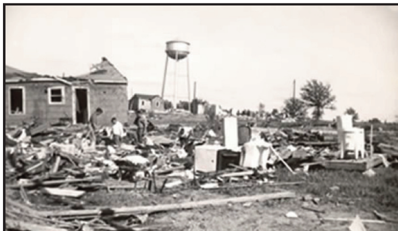
Figure 2.3.2: Flint Tornado Destruction 2 Source: Flint Public Library
