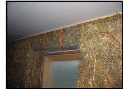
FIGURE 21: Interior Insulation; Source: http://strawbalefarms.com/about.html
