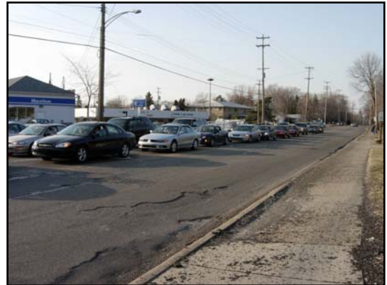
Photo 8: Example of Sidewalk Quality on
