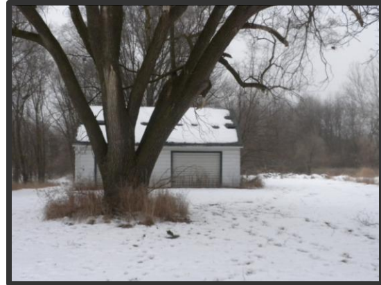
Figure 3: Garage on site
