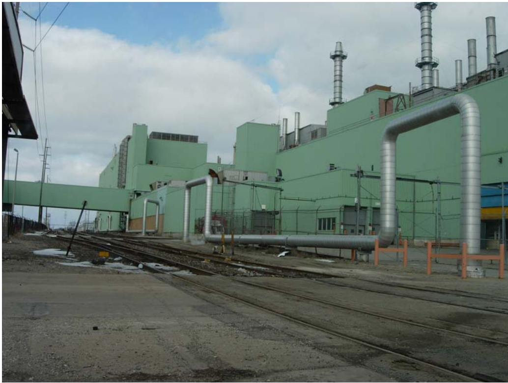
Looking at GM Plant #6 from Southwest Corner
