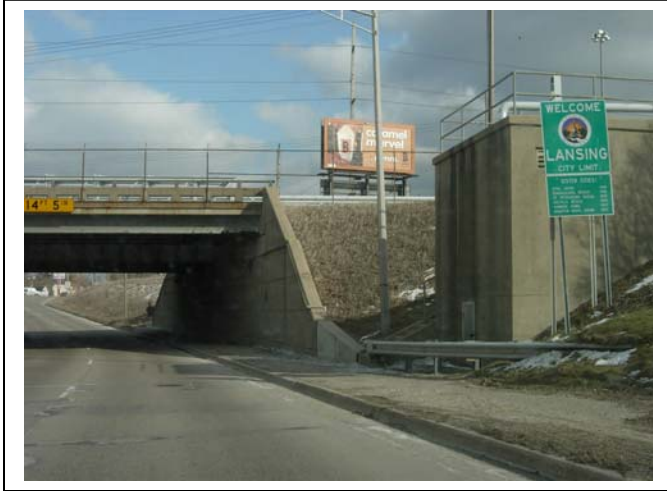
Figure 4.6: View of the Verlinden Avenue Site from Saginaw Street
