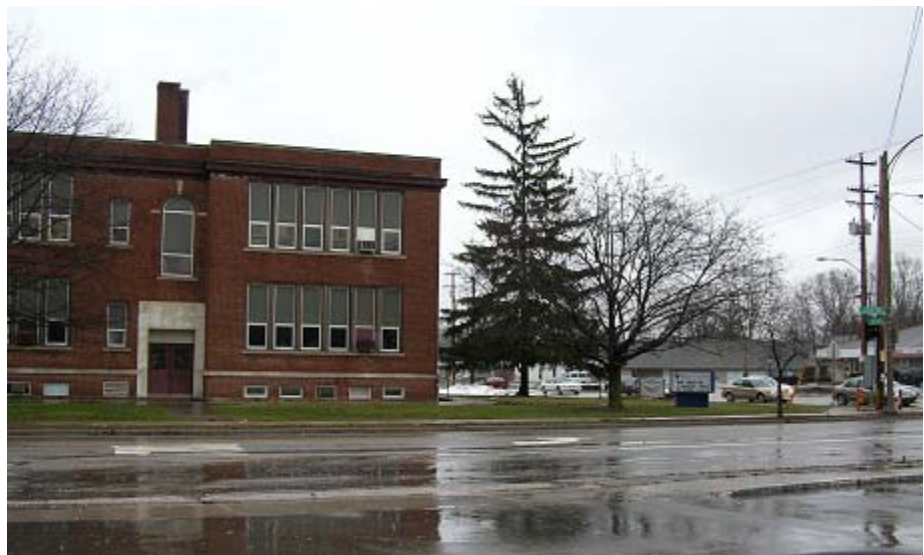
A view facing New City Academy, a charter school located at the Northeast corner of Holmes and Pleasant Grove.
