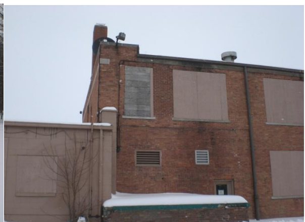
Figure 4.35: Vacant School Building
