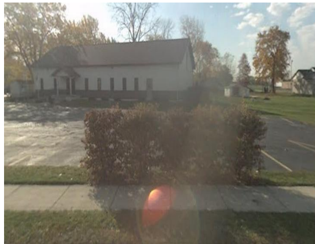
Figure 4.26 Church in Block 8
