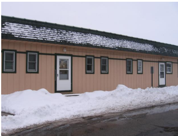
Figure 4.7: Vacant Building in Block
