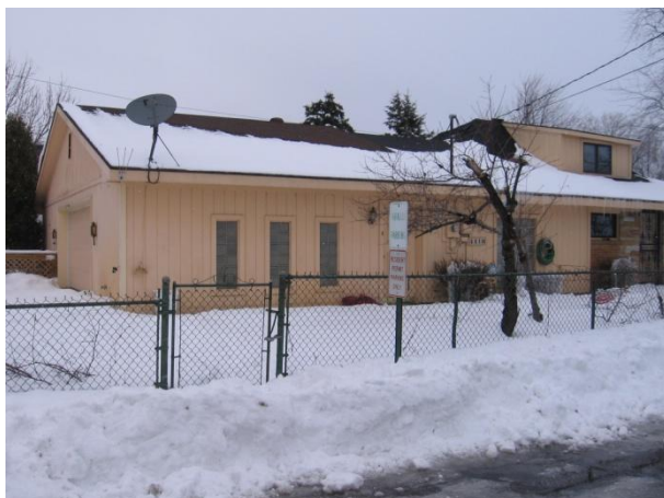
Figure 4.10 Housing in Block 3
