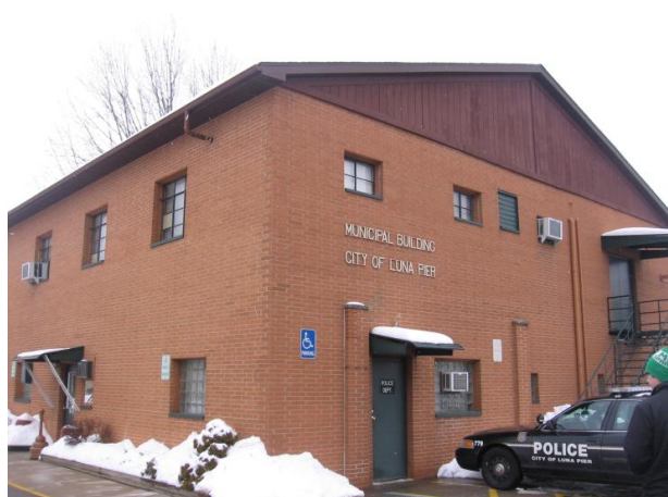
Figure 4.4: Luna Pier City Hall in Block 1
