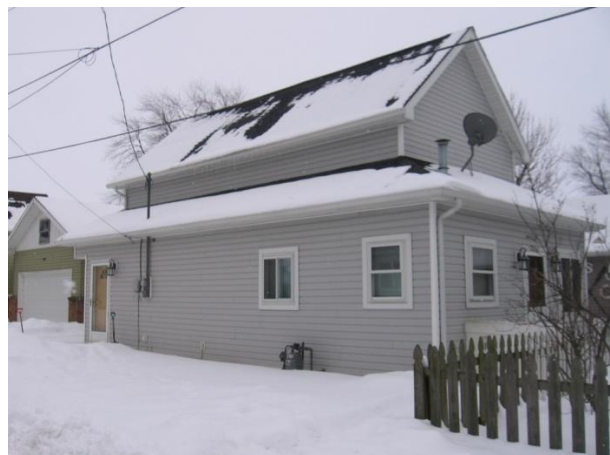
Figure 4.11 Housing in Block 3
