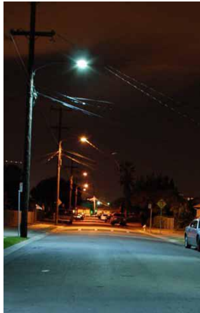
FIGURE 3.3: Street View of LED lights
