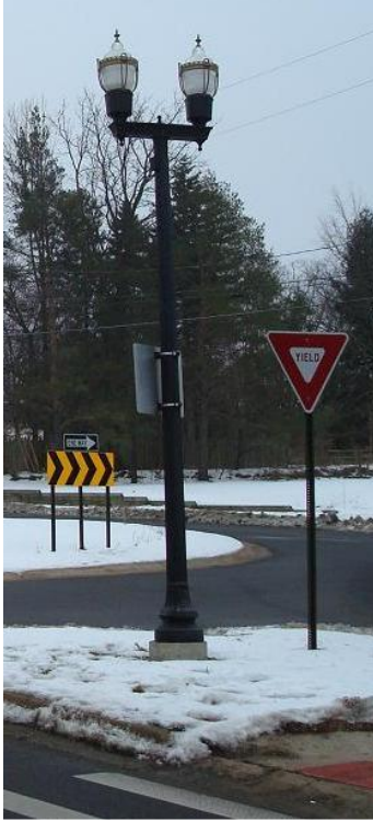
FIGURE 1.30 Existing Traditional Streetlight at the Hamilton Roundabout
