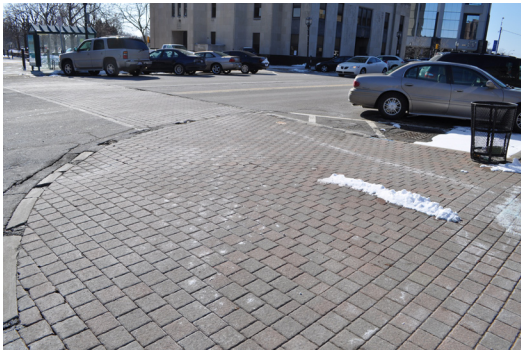
Figure 3.14 Pedestrian Bump out
