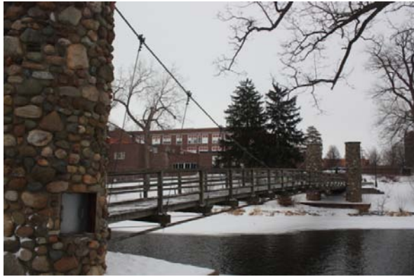
Figure 8: Bridge across the Shiawassee River
