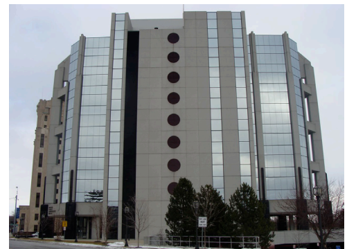
Figure 2.6 Macomb Co. Admin. Bldg
