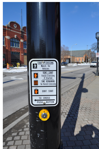
Figure 3.17, Pedestrian Actuated Crosswalk Signal
