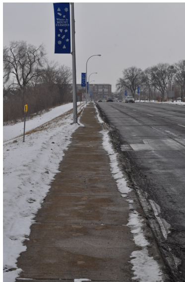
Figure 3.8 Narrow Sidewalk and missing pedestrian buffer.
