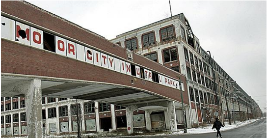
Figure 3: Packard Plant Detroit, MI
